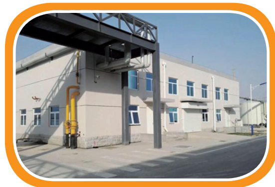
鍋爐房 Boiler room
